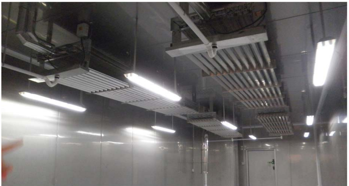
Evaporador ECT com apara pingos ECT coil with drip tray
