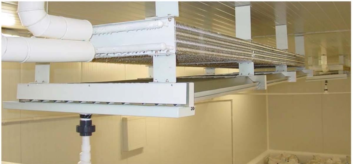
Evaporador ECT com apara pingos ECT coil with drip tray
